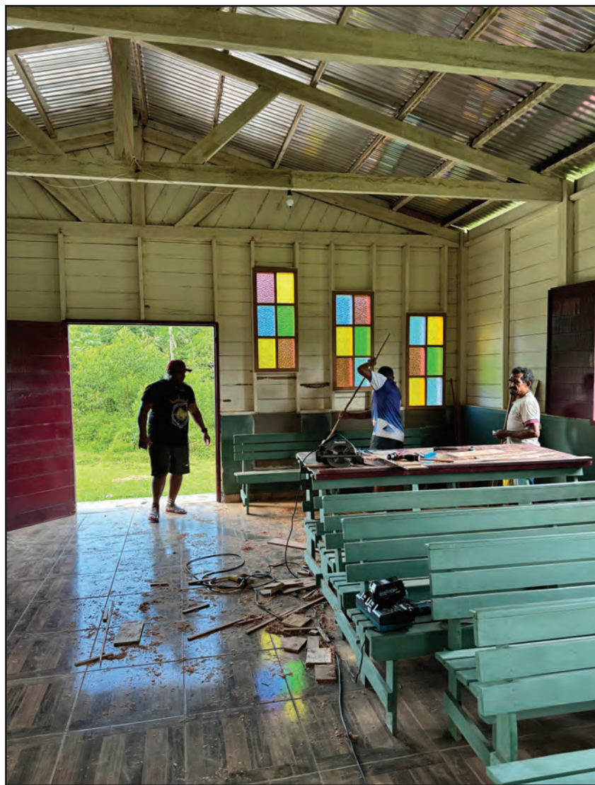
Building "stuff" at the mountains on the Moa River.
